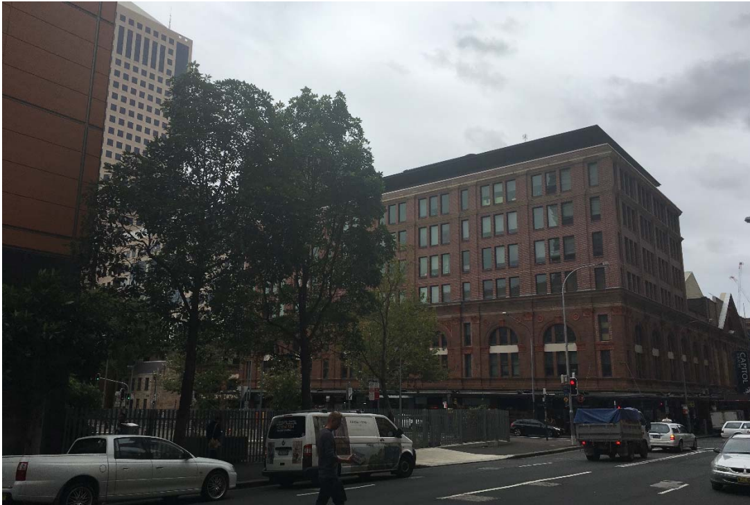
Figure 3: Looking west across the subject site to the Manning Building
