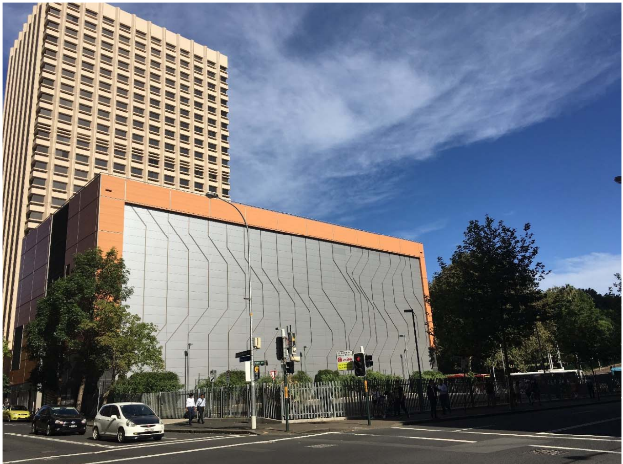
Figure 2: The subject site as viewed from the corner of Campbell and Pitt Streets, with the Belmore Park substation located to the east of the site
